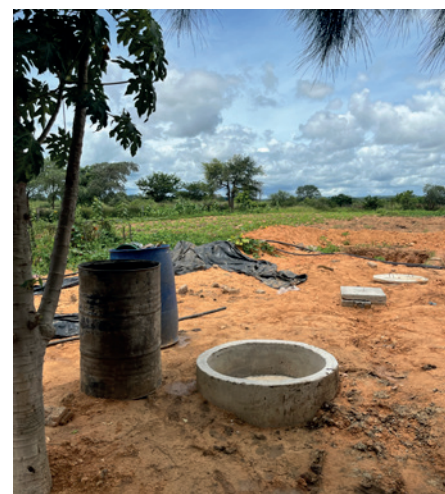
A recently installed biodigester
